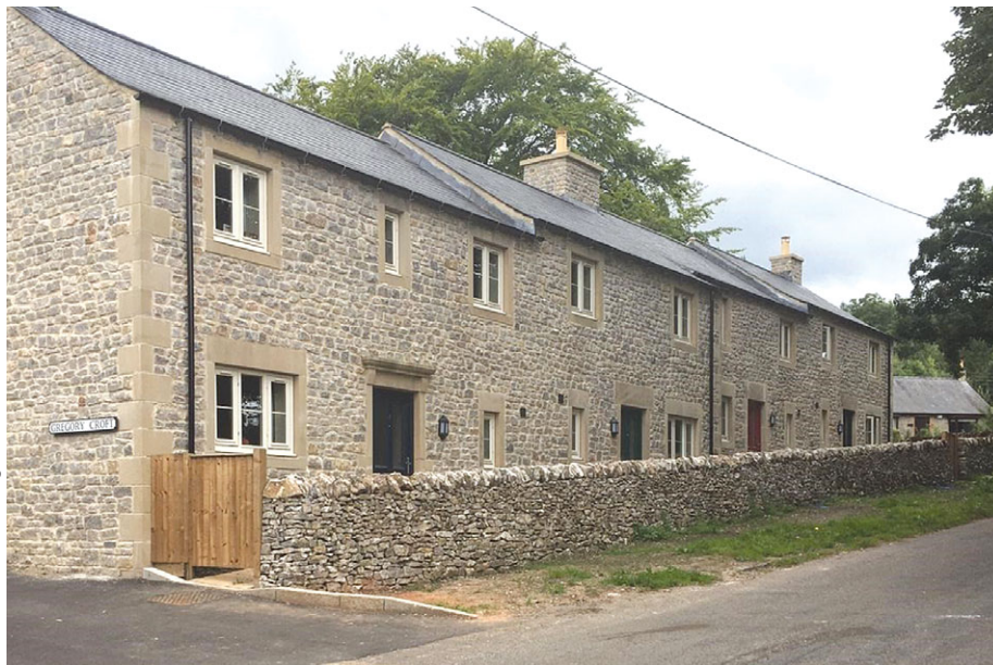
New affordable housing by Peak District Rural Housing Association, Taddington, Derbyshire
