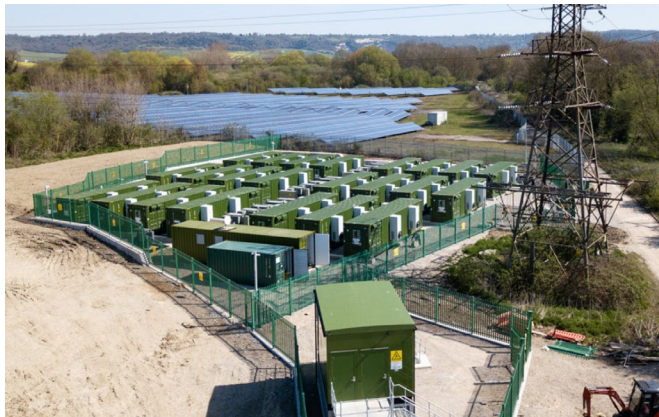
Grid scale battery storage
