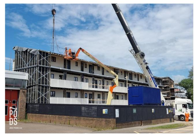
Picture: Making of "Fortis House" by using volumetric offsite construction methodology
