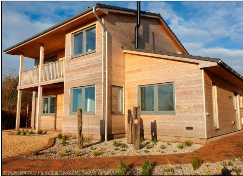
Project by Mitchells Construction & Development Ltd, FMB Southern Counties
